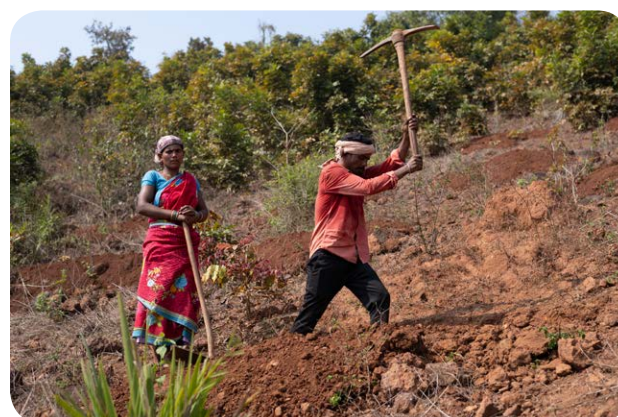
Residents dig staggered contour trenches (SCTs) as part of watershed work
